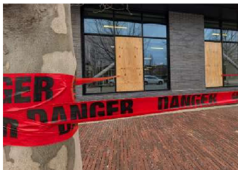
Broken windows at The Forge. From The B Square Bulletin. April 2025.
