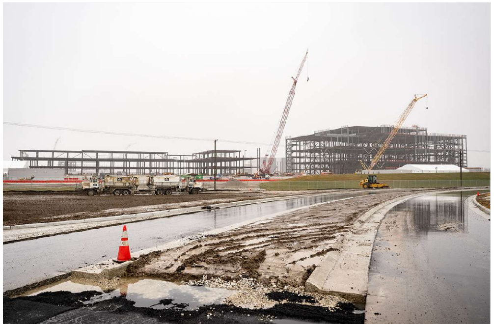
Eli Lilly construction at the LEAP District
